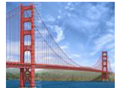
Golden Gate Bridge
